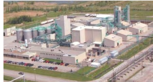
20 MW PEM H2 Production Expansion in Quebec (Source: Air Liquide)
