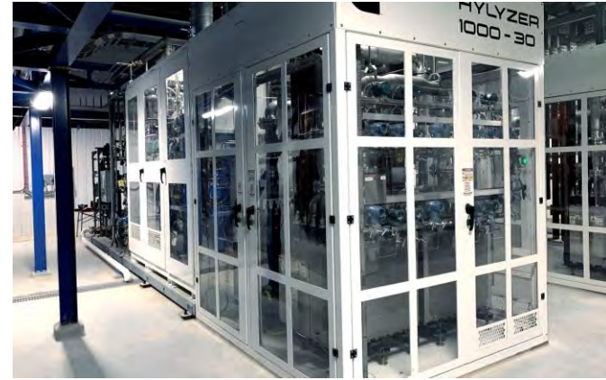
Cummins PEM Electrolyzer (Source: Cummins)
