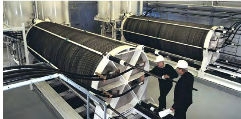
NEL Alkaline Electrolyzer (Source: pv-magazine)
