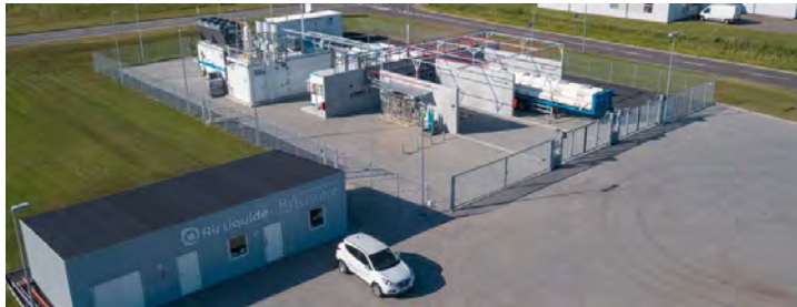
1.2 MW H2 Production + TT Filling in Denmark (Source: Air Liquide)
