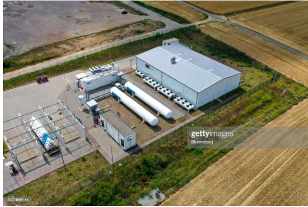
6 MW H2 Production + TT filling & NG Blending in Germany (Source: gettyimages)
