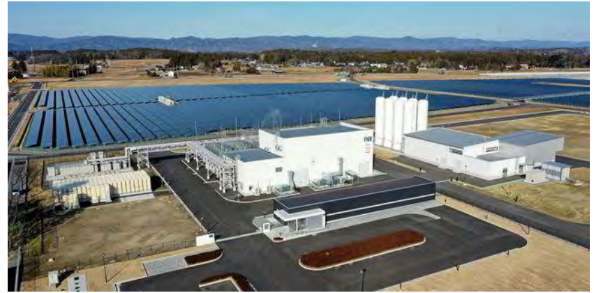
10 MW H2 Production + 20 MW Solar Farm in Japan (Source: rechargenews.com)
